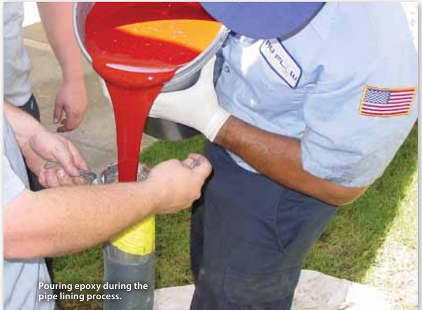
Pouring epoxy during the pipe lining process.
