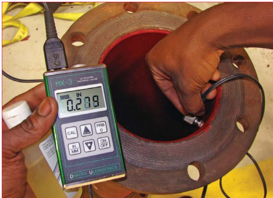
Technicians used a micrometer to check the thickness of the finished liners.
