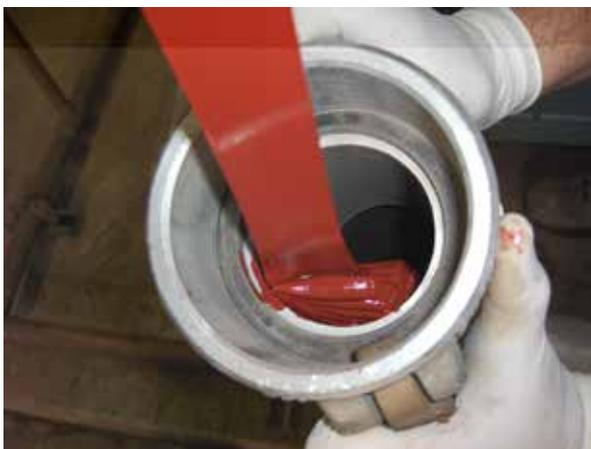
The epoxy is blown through the pipe system to create an even coat, which will cure (aka: dry) and create a protective liner.
