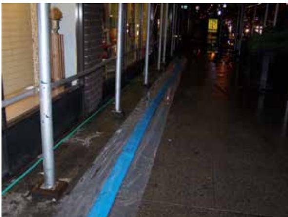
Technicians push the Nu Drain epoxy through the structural liner. Once completed, the liner can be inserted into a pipe line to create a protective liner.
